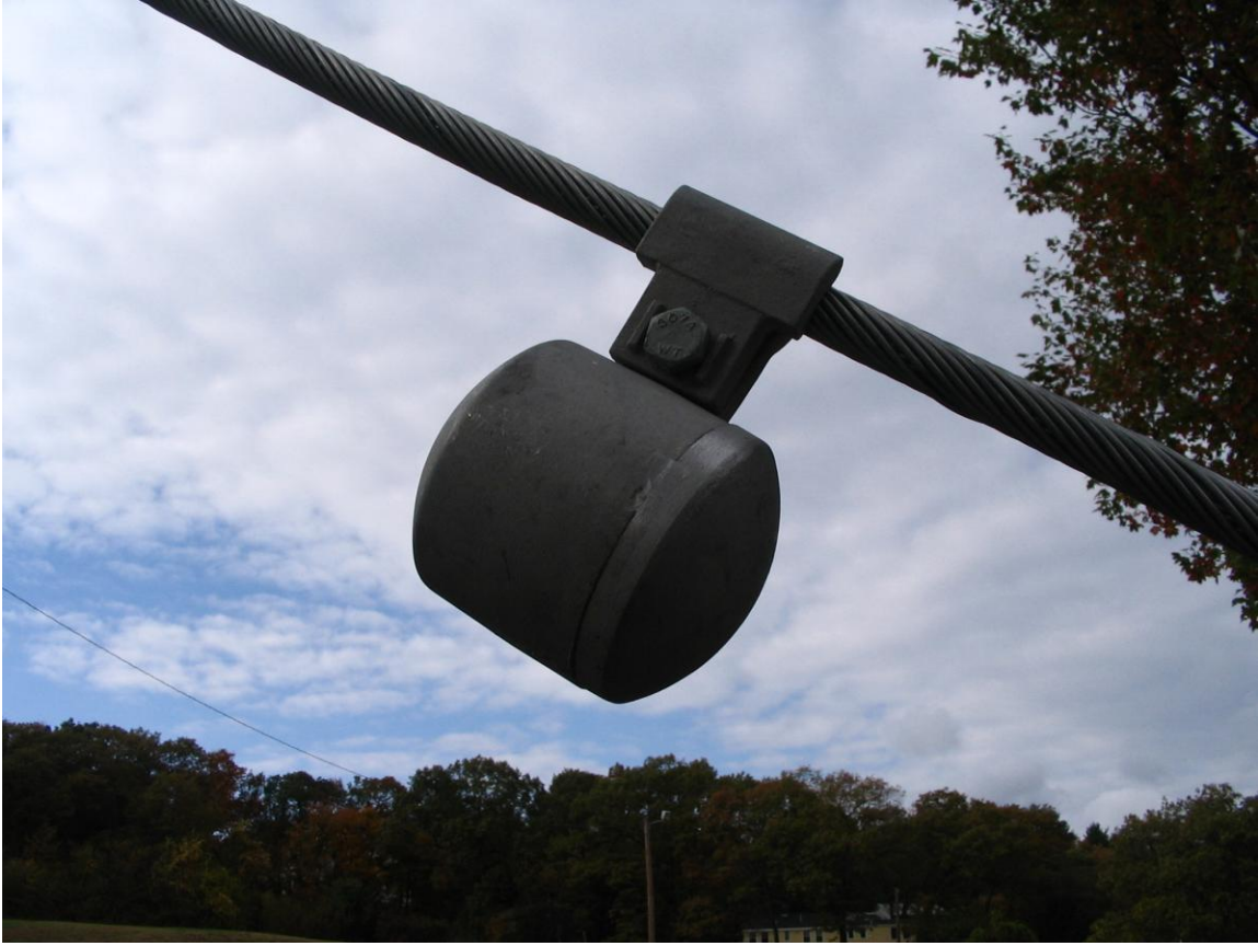
Photo #3 Mod IX AR DAMPER on guy cable
