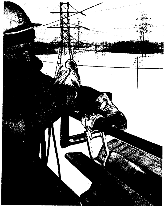
Crew member is shown installing Windamper anti-galloping device on line. Study indicates the 15-year old device still offers the most economic protection.
