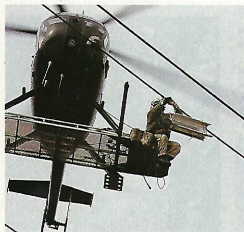
4. Anit-galloping device (right) is constructed of aluminum and sized for the conductor diameter and length of span. Weight is up to 33 lb
