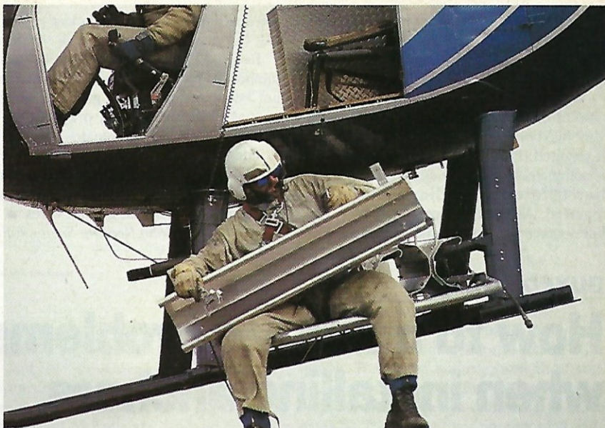
5. Helicopter is electrically bonded to the transmission line for all hot-line installations (left)
