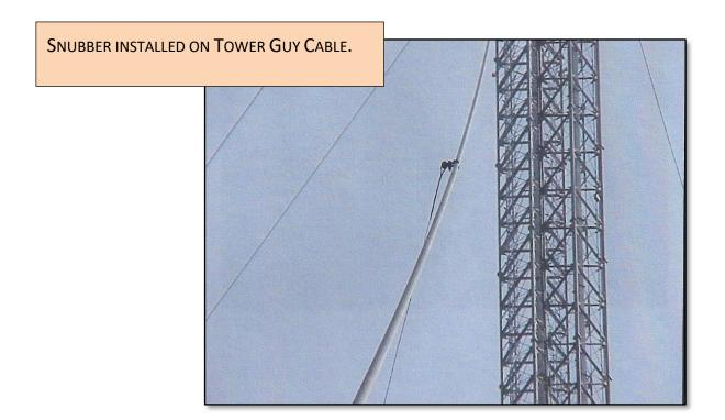
AR Snubber Systems are anti-galloping dampers. Installed horizontally on the guy cable, the Clamp can rotate towards the ground up to 90 degrees. This twisting action helps arrest the galloping motion.
